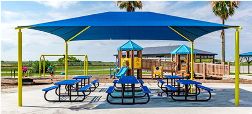
Figure 1 Outdoor Shade Structures
